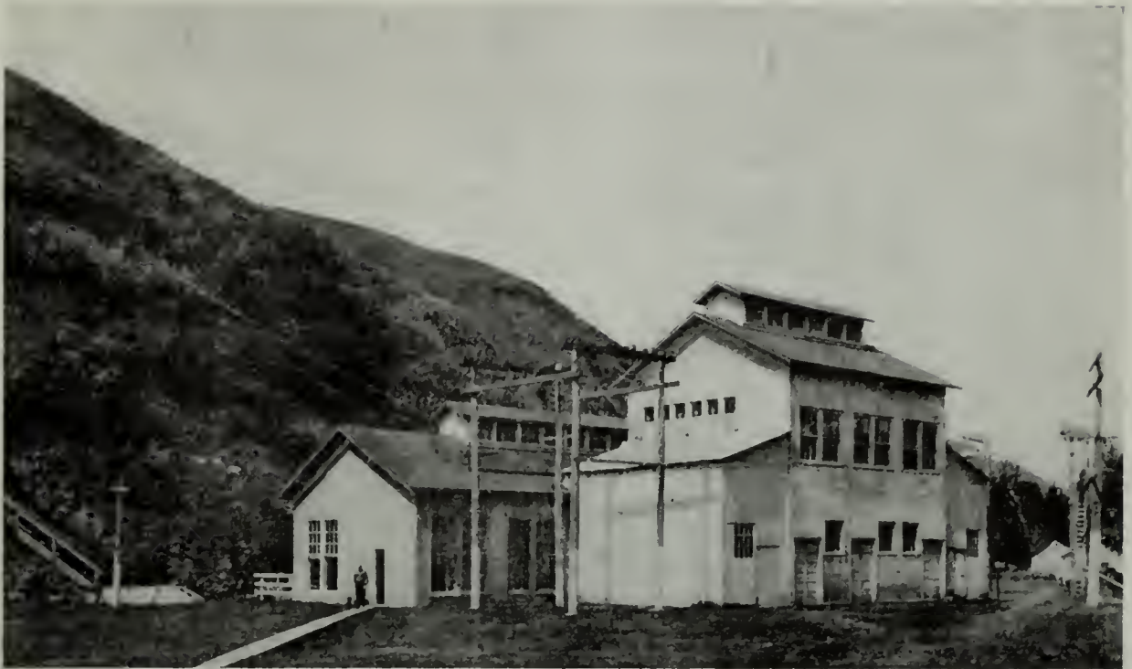
Walla Walla River Generating Station - July, 1910
